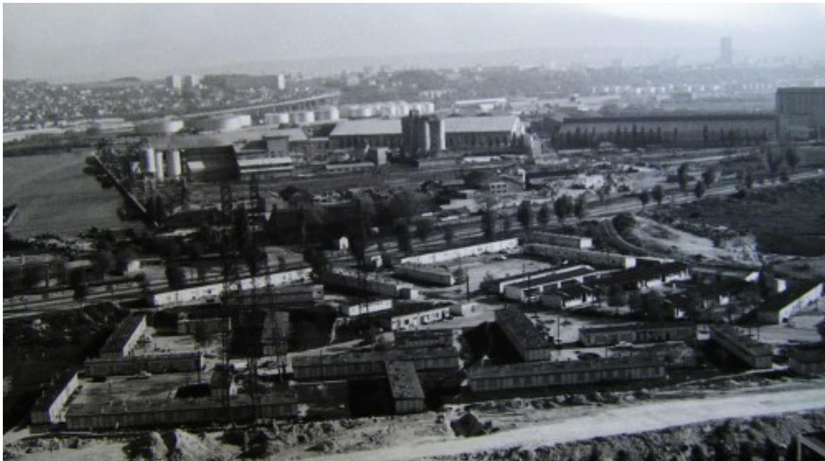
Bird's-eye view of Cité 51, along the main road through the Port of Gennevilliers © M. Hervo
